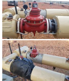
Back Pressure Valve Before & After
